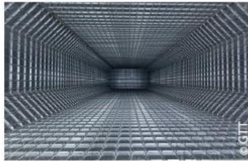
Storage tank for seaborne transport of LNG
